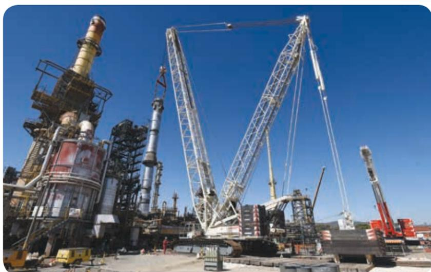
*At the Chevron refinery in the Western Cape, MegChem was the engineering contractor for four major upgrades at the refinery: the fluid catalytic cracking unit (FCCU), replacing the Texas tower and the crude column, and for a fast track project to implement the required plant changes in order to produce 50 ppm diesel.*
